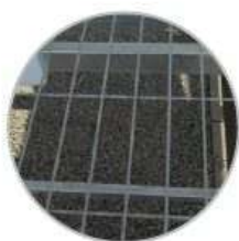
Welded wire mesh top
